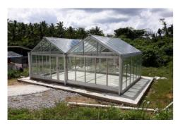
The invention of a Greenhouse Solar Dryer uses solar energy to generate heat for drying purposes, with features such as ventilation, temperature control, and even drying. BBC provides training and technical support to users, as well as research and development to continuously improve the efficiency and effectiveness of the dryers.
