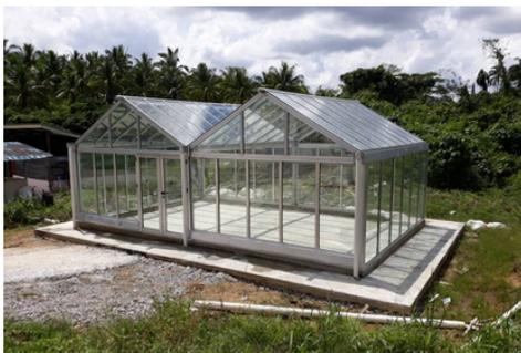
The invention of a Greenhouse Solar Dryer uses solar energy to generate heat for drying purposes, with features such as ventilation, temperature control, and even drying. BBC provides training and technical support to users, as well as research and development to continuously improve the efficiency and effectiveness of the dryers.
